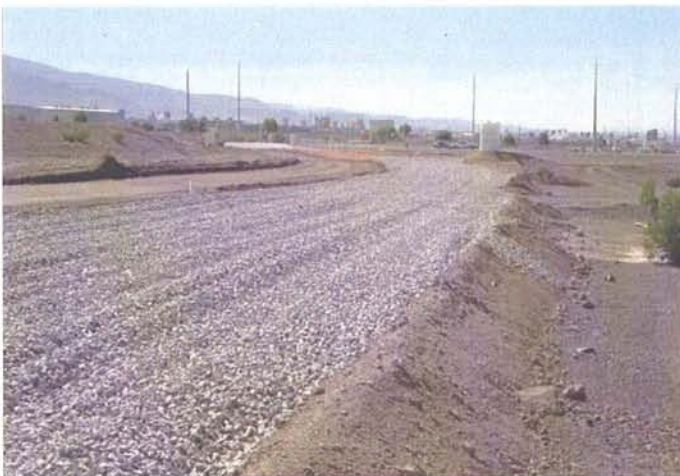
Eastside: Egress 1" cap rock approaching decontamination pad. Installed to assist in decon.of tires.
