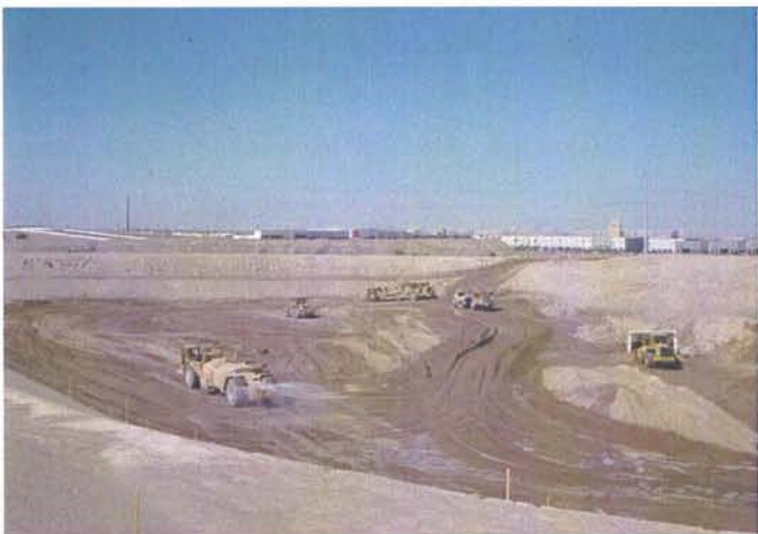
CAMU: Phase 2, placing lift of soil on floor, with dust control..
