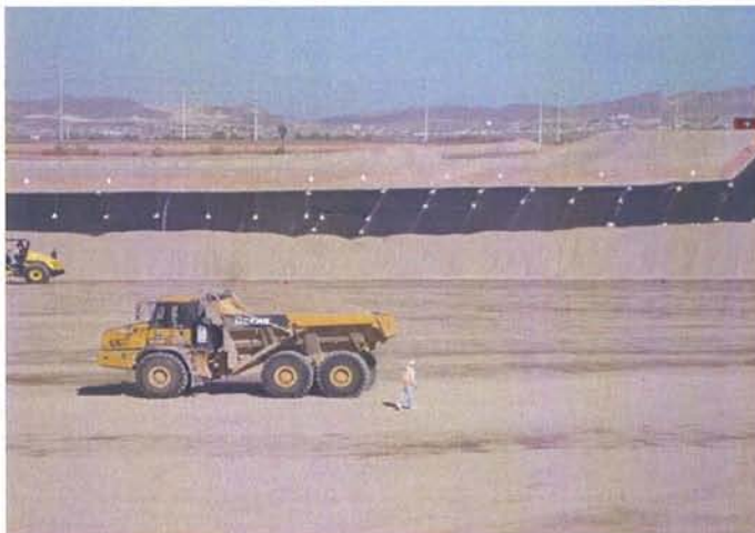
CAMU: Phase 1 Geosyntec monitoring proof rolling of lift with a loaded 40 ton haul truck..
