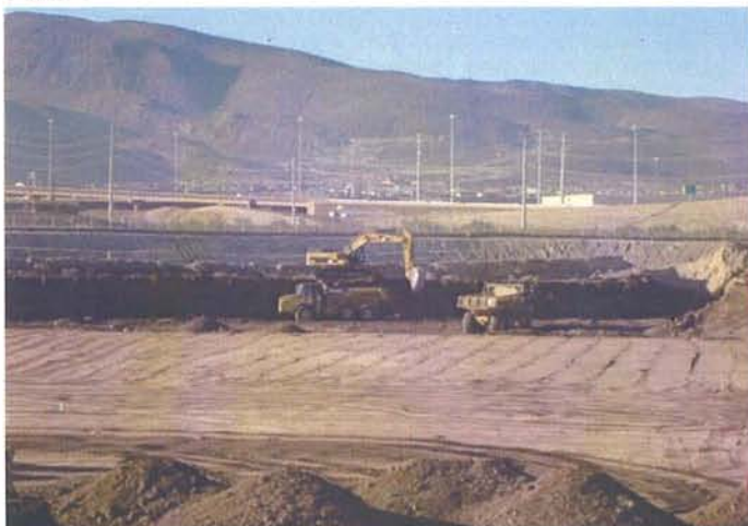
CAMU: Western Ditch Soils, placed and rolled
