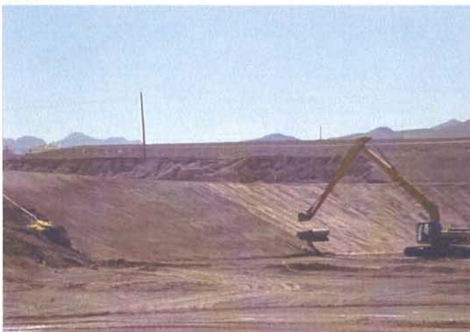
CAMU: Phase 2, east slope being rolled. Preparing for liner
