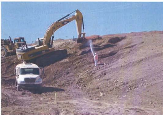
CAMU: Phase 2. Western ditch grading slope. With dust control.
