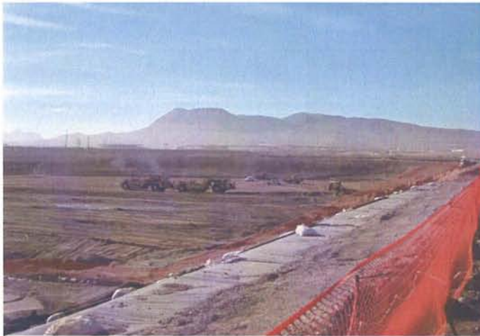
CAMU: Phase 2. scrapers removing clean soils.
