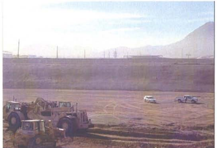
CAMU: Phase 2, Scrapers removing clean soil. Subgrade and southslope preparation.
