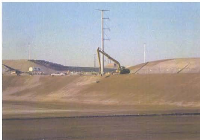
CAMU: West slope of Phase II being rolled with long stick excavator and roller attachment.
