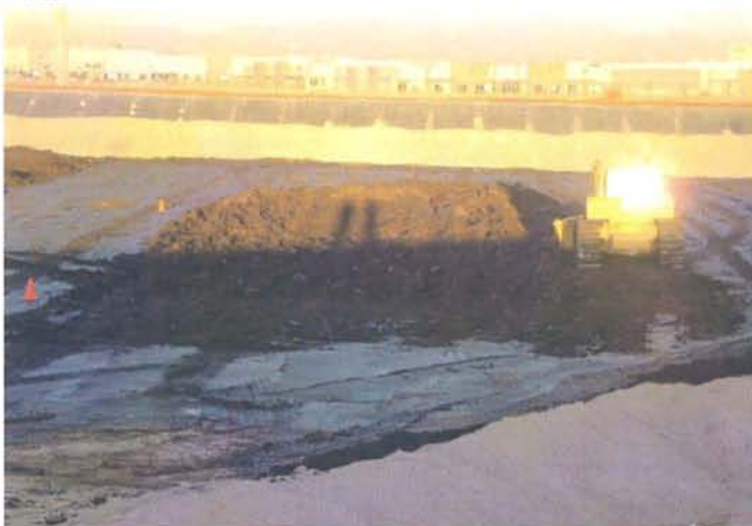
CAMU: Phase I area failed proofrolling test. Being reworked.
