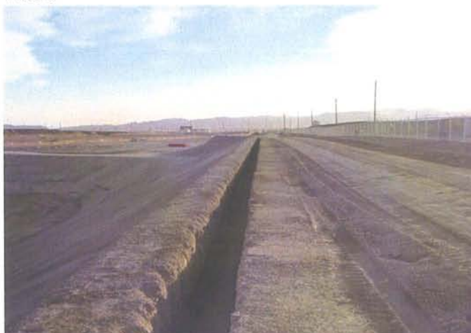
CAMU, Phase II, Anchor trench south end.
