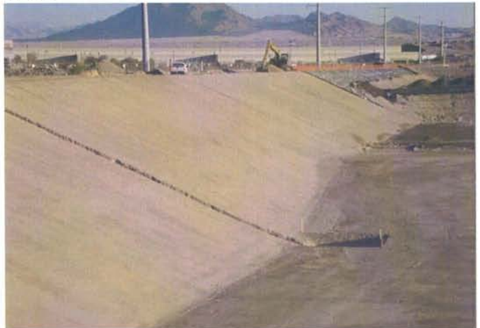
CAMU: Phase II, Sump and riser trench excavated.
