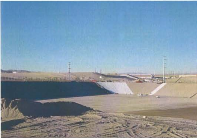
CAMU: Phase II, Southwest Liner installation continues.
