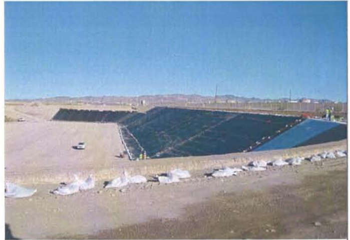
CAMU: Phase II, liner installation, beginning the southwest corner.
