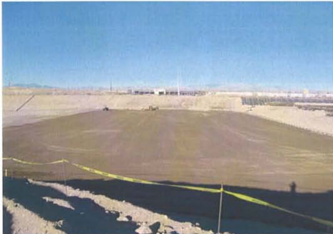
CAMU: Western ditch floor and west slope final grading and rolling..
