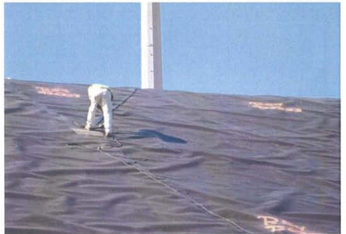
CAMU: Phase II liner installer.
