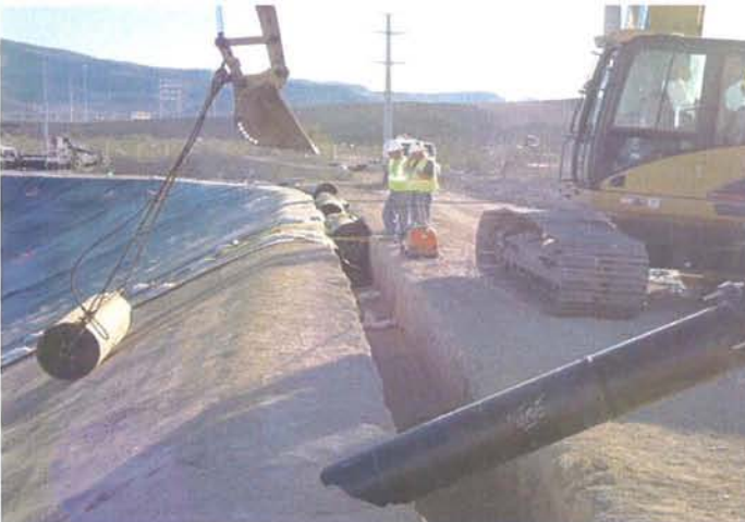
CAMU: Phase II, West slope rerake and roll after pipe installation.
