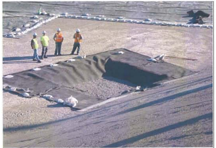
CAMU: Phase II, Vadose zone monitoring sump installed.
