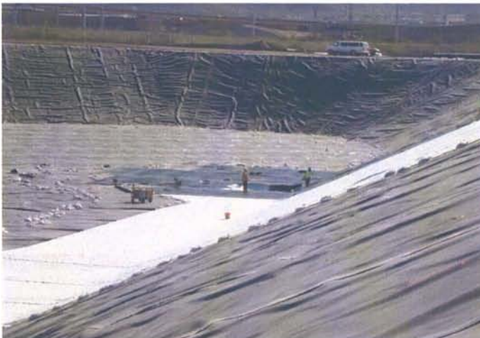
CAMU: West slope and sump liner installation.
