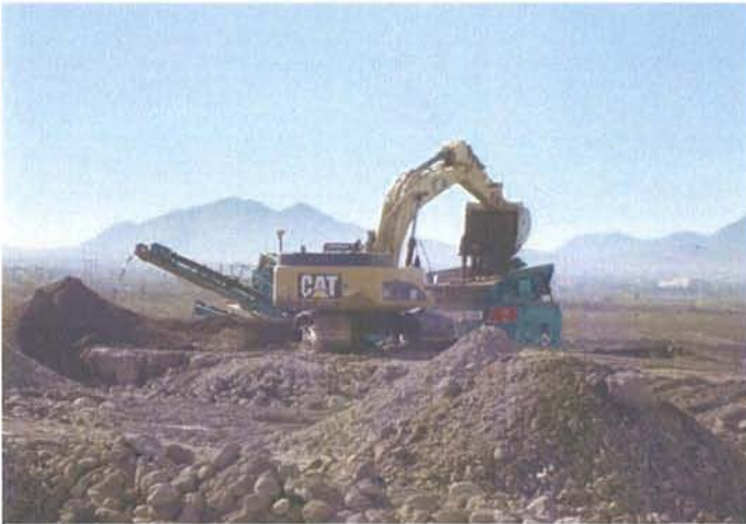
Eastside: PUA-4 powerscreening moisture conditioned soils
