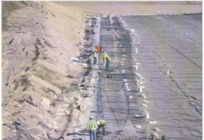
CAMU: Phase I & Phase II tie-in of liner.
