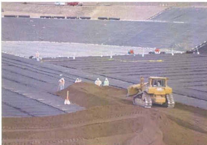
CAMU: Operation Layer pushing out east parallel with LCRS pipe system. Watching oversight is Entact, Geosyntec and Weston.
