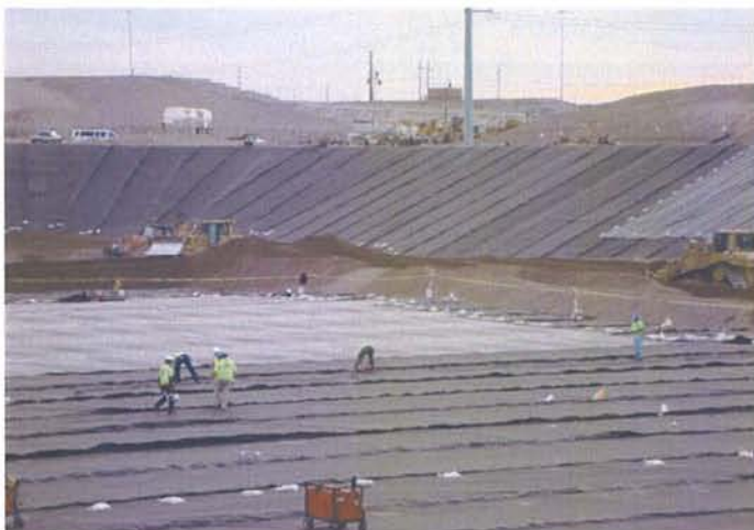
CAMU: Phase II, Geocomposite installation and operations layer grading.
