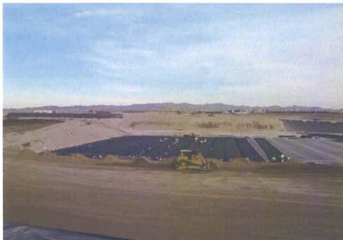
CAMU: Phase II operation layer grading for night shift.
