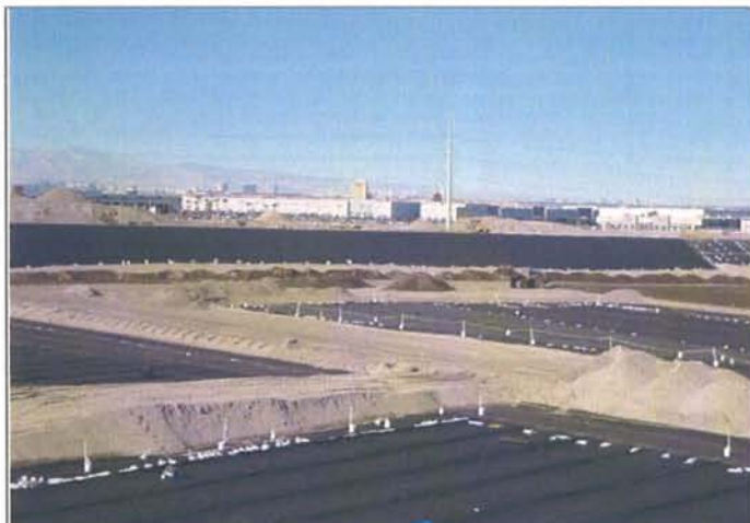
CAMU: Phase II, operations layer, finger roads to support toe drain installation.
