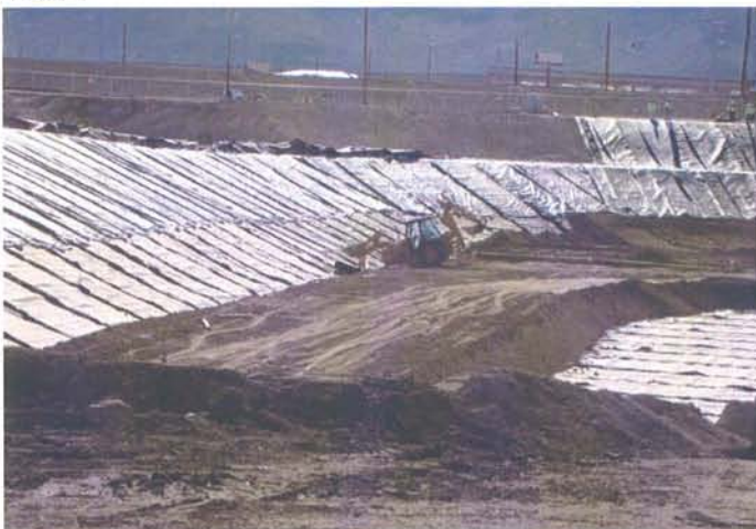
CAMU: Phase II East slope, toe drain rock installation.
