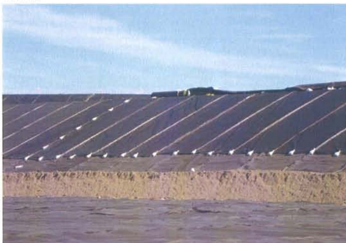
CAMU: Phase II East slope operations layer road for toe drain installation.
