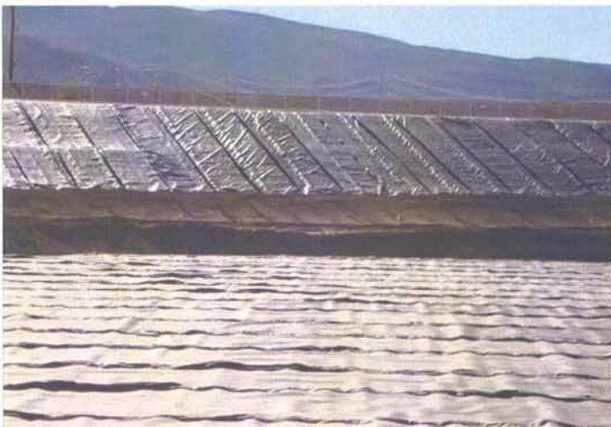
CAMU: Phase II, Operations layer placed on slope.
