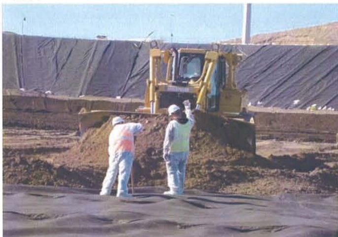
CAMU: Phase II, Operations layer placement monitored by Entact, Geosyntec and Weston.
