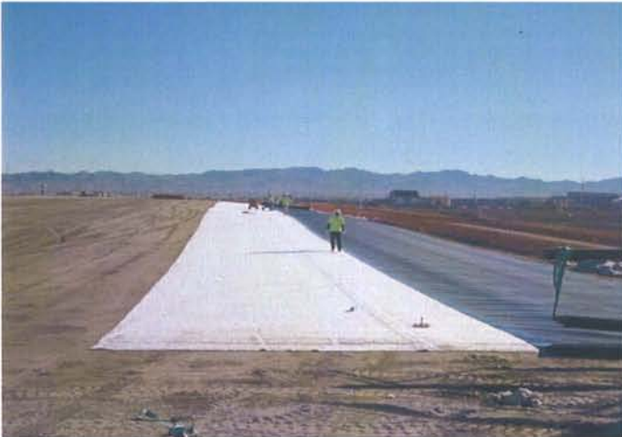
BMI North Landfill: Beginning of geosynthetics installation south end.
