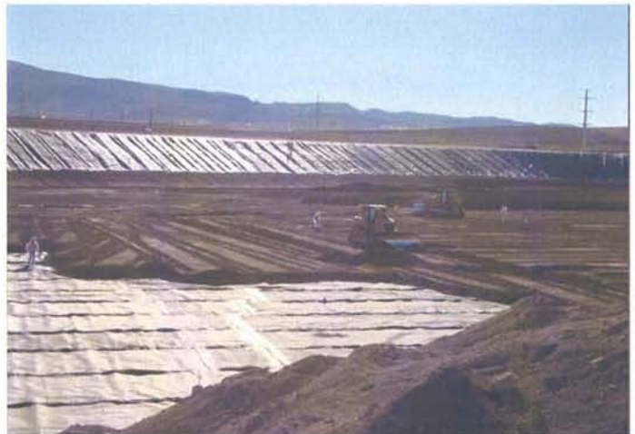
CAMU: Phase II, Operations layer grading.
