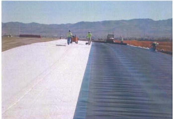
BMI North Landfill: Beginning of geosynthetics installation, south end.
