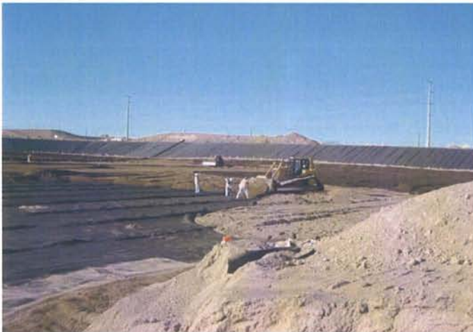
CAMU: Phase II operations layer installation.
