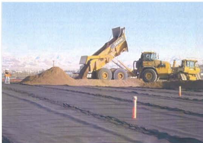
CAMU: BMI Landfill North, First lift push-out
