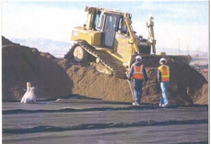
CAMU: BMI Landfill North, First lift push-out.
