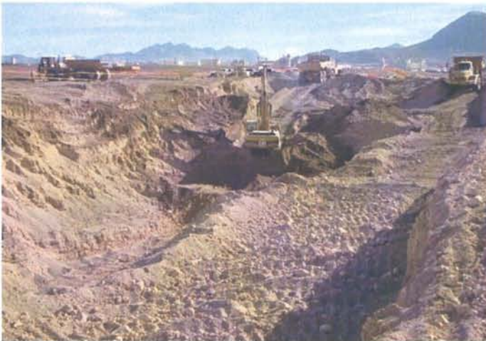
CAMU: NW Basin/Phase IIIB trench excavation.
