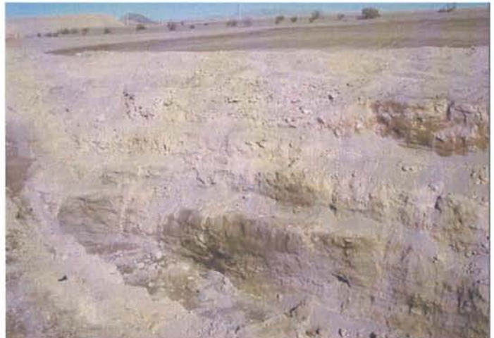
CAMU: NW Basin/Phase IIIB trench excavation east wall showing more discolored soils to be removed
