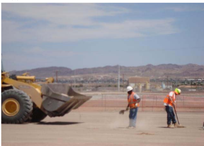
CAMU: BMI South Landfill subgrade preparation.
