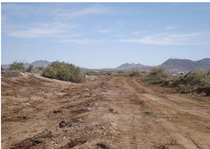
Western Hook: Ditch, clearing and grubbing.
