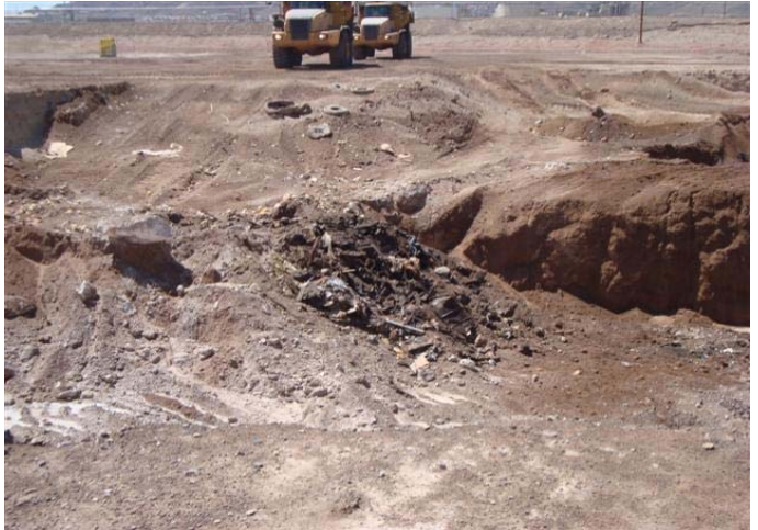
CAMU: SW-1 - SE-1. additional waste found beyond design limits.
