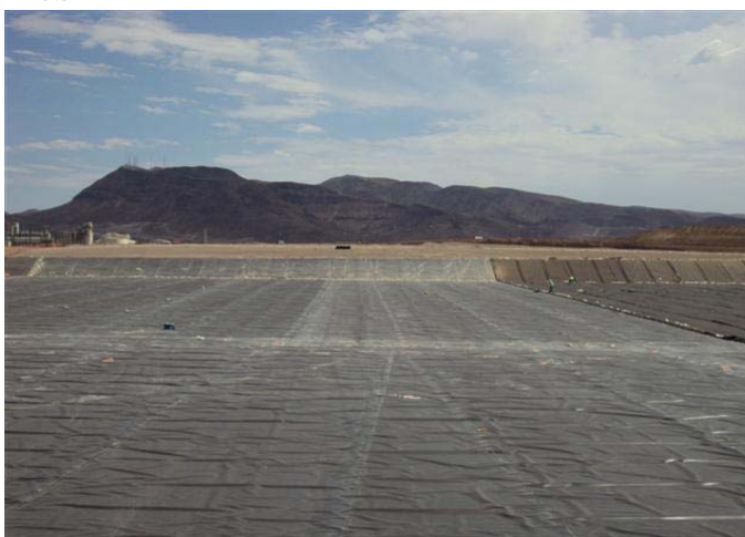
CAMU: Phase IV Liner installation.
