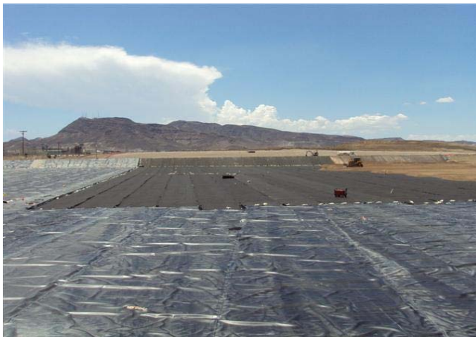
CAMU: Phase IV, liner installation.
