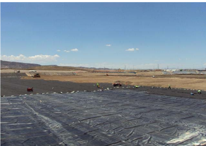
CAMU: Phase IV, Liner installation..
