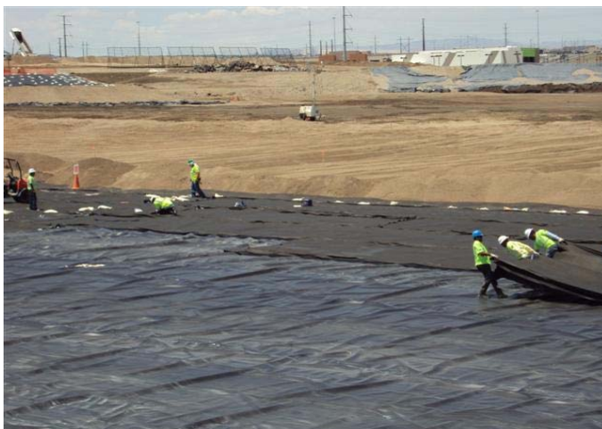
CAMU: Phase IV Liner installation.
