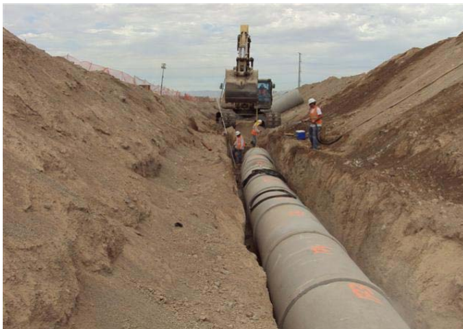
CAMU: RCP, Stormdrain system installation.
