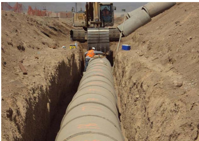
CAMU: RCP, Stormdrain system installation.
