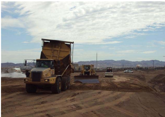
CAMU, Phase V, SE-1, slit trench backfill.
