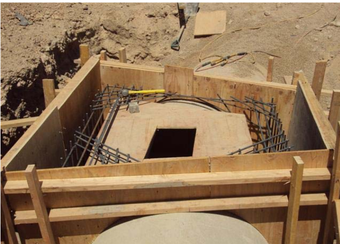
CAMU: 42" RCP storm drain system, manhole #1.
