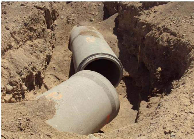
CAMU: 42" RCP storm drain system. To be manhole #2.
