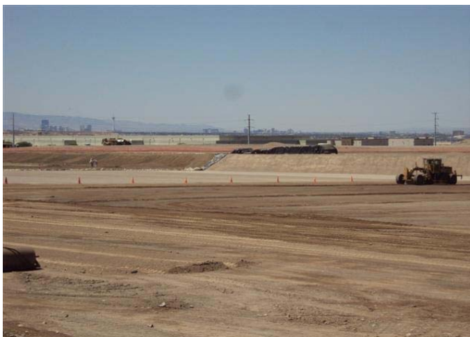
CAMU: Phase V, subgrade preparation.
